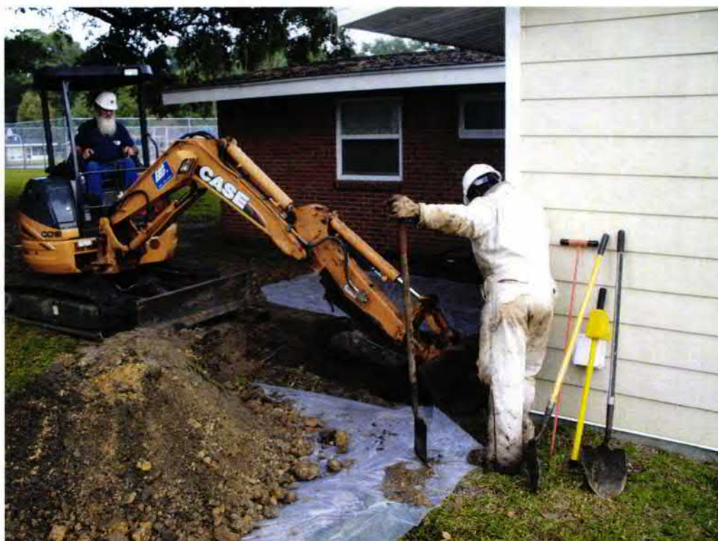
Picture 2: UST 454Elderberry excavation in progress .
